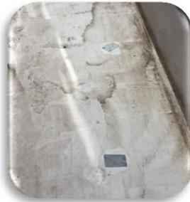
*Phase 2 – Hole in the roof patched up*
